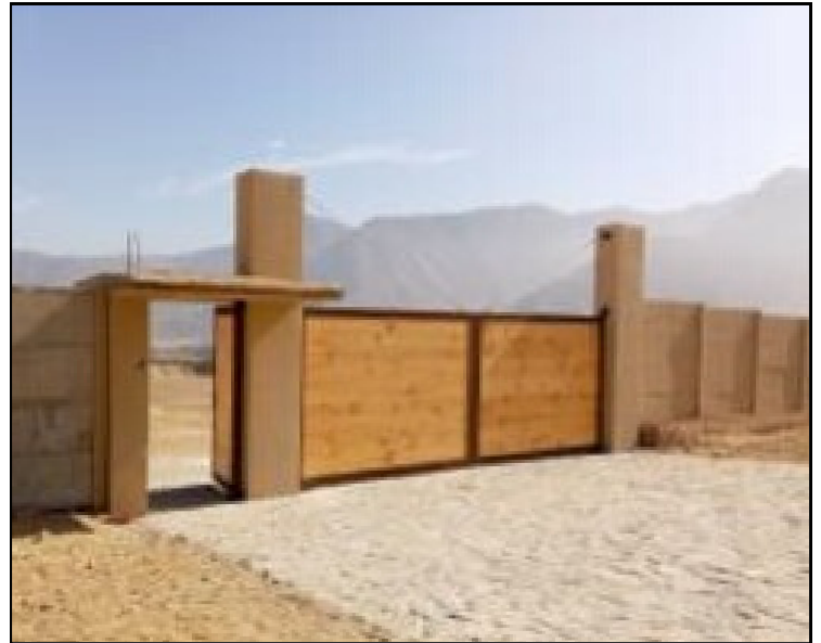
Photo: New perimeter wall at Dhamma Suriya, Peru.
